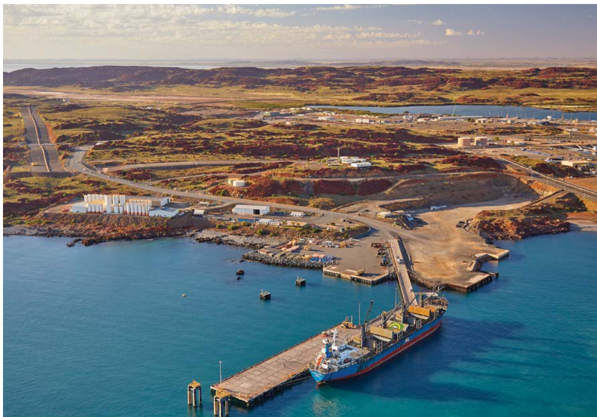
The existing Dampier Cargo Wharf.
