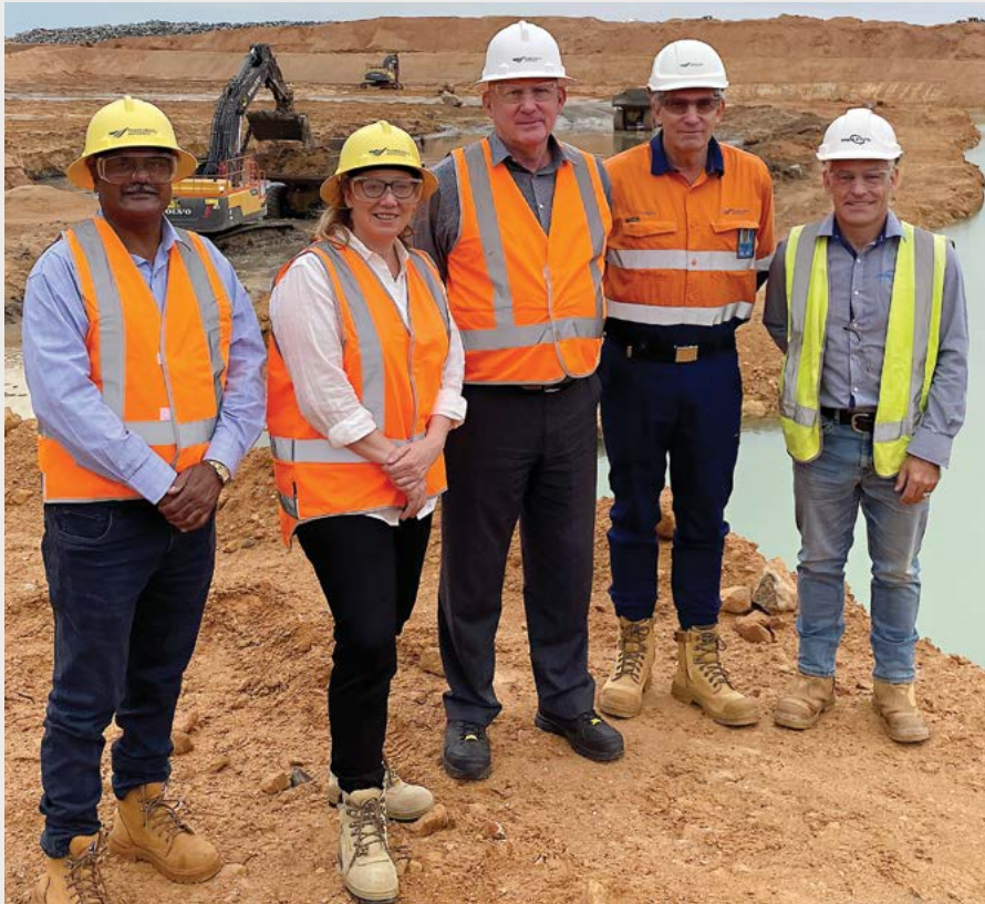
Member for Pilbara Kevin Michel, Minister for Ports Rita Saffioti, the Authority's CEO Roger Johnston, General Manager Engineering and Infrastructure Charles Kretzmann and MGN Civil Project Manager Guy Schweitzer toured the Spoilbank Marina construction site in April.
