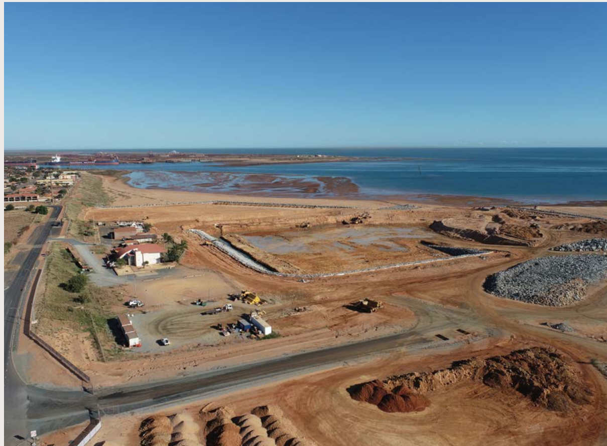
The Spoilbank Marina work site in June 2022.
