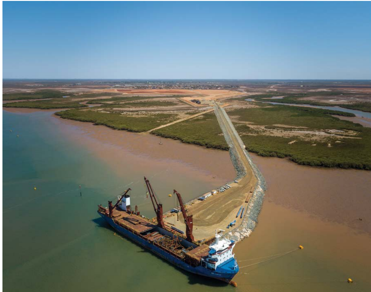
A vessel at Lumsden Point Module Offloading Facility in October 2021.
