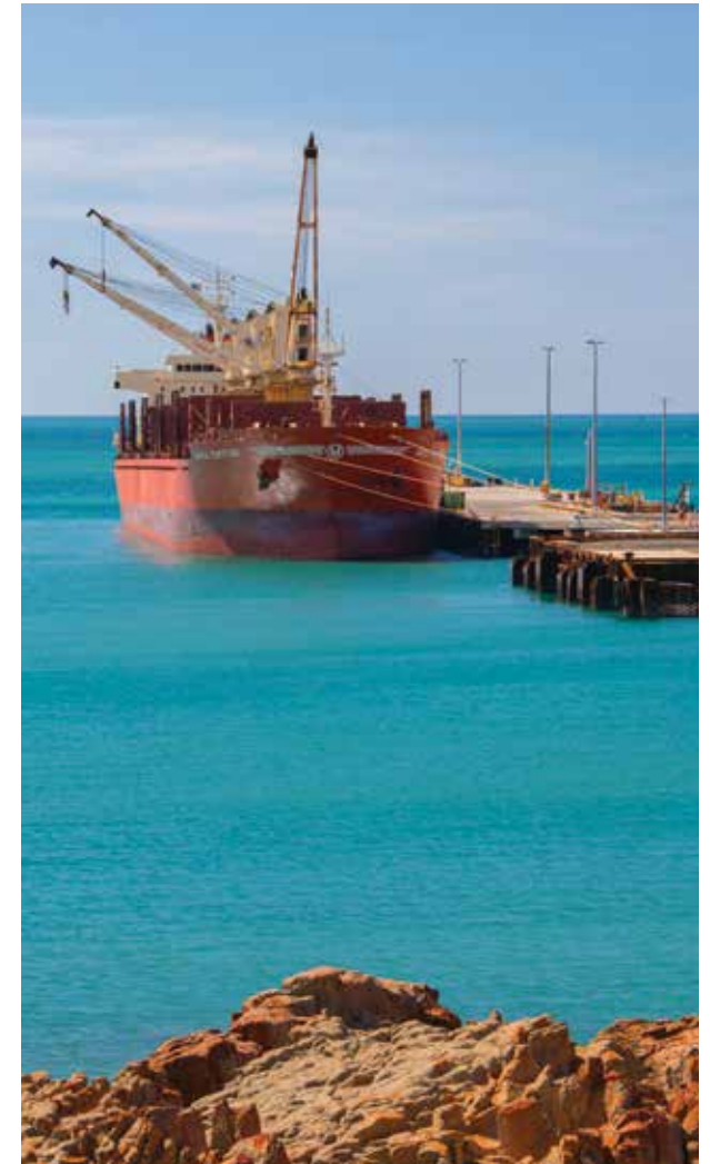
Dampier Cargo Wharf at the Port of Dampier.
