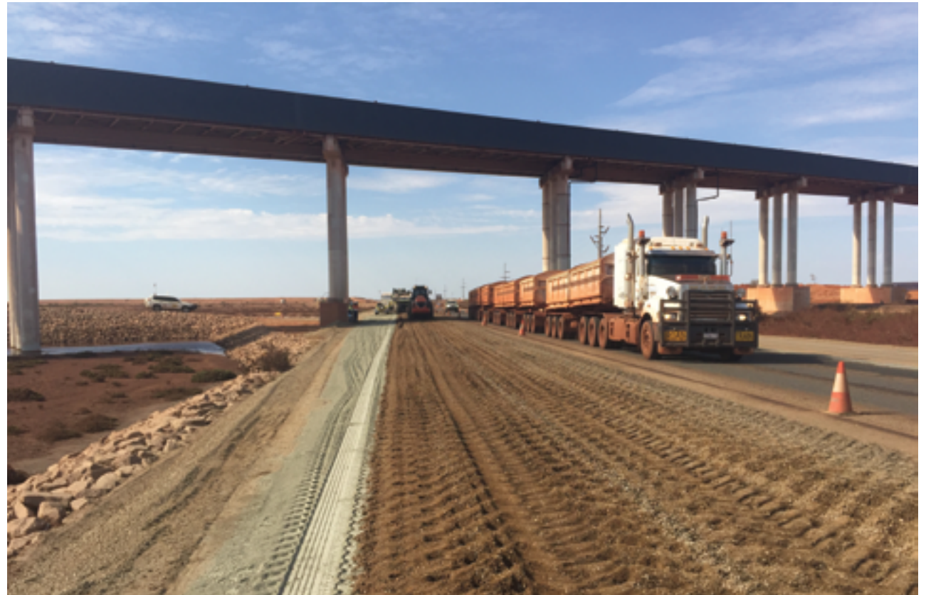
Rehabilitating Utah Road, Port Hedland
