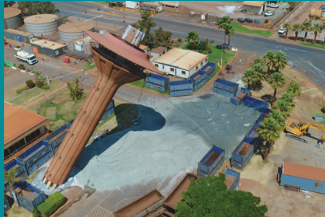
Felling of the Port Control Tower at the Port of Port Hedland
