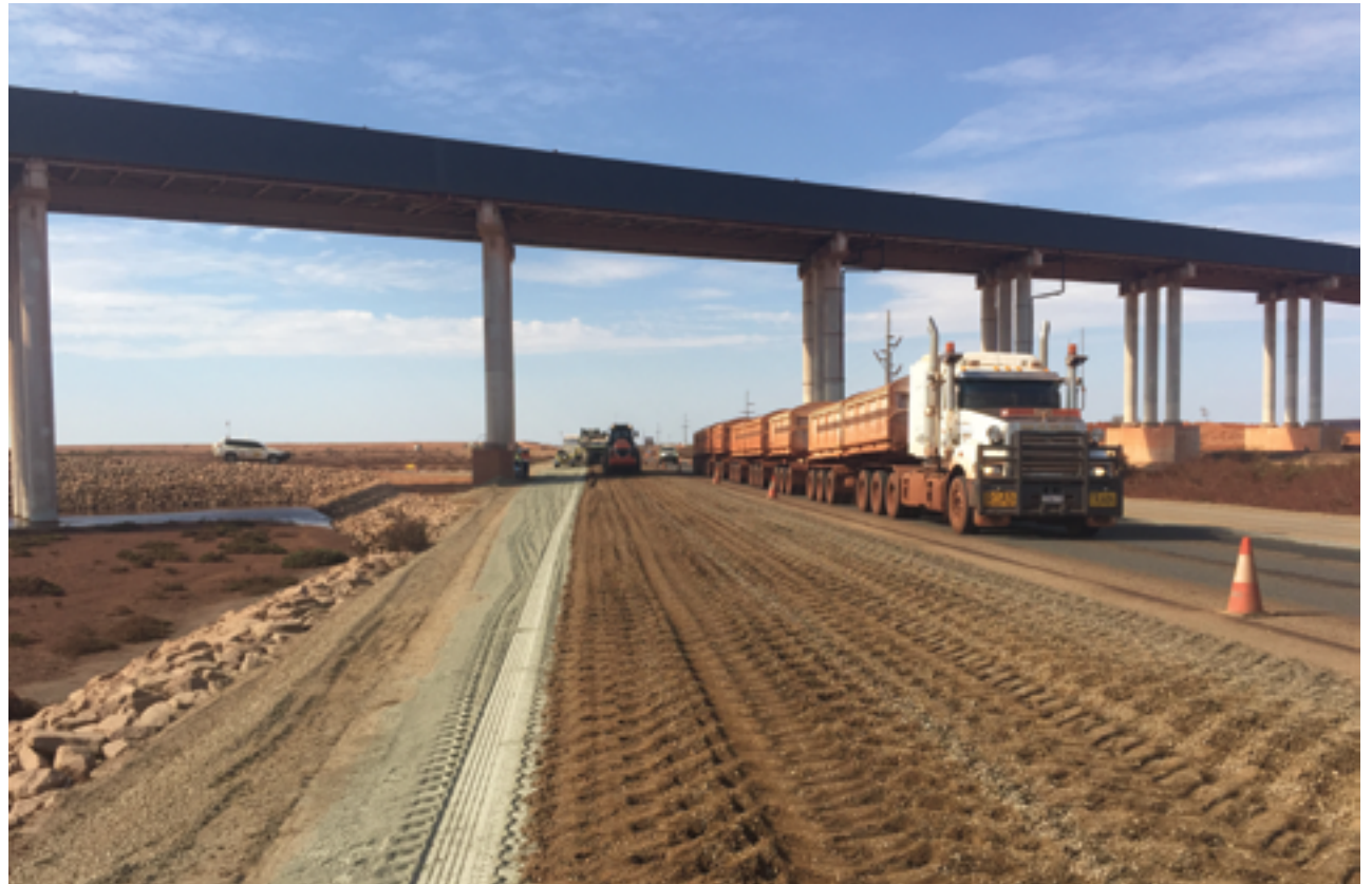
Rehabilitating Utah Road, Port Hedland
