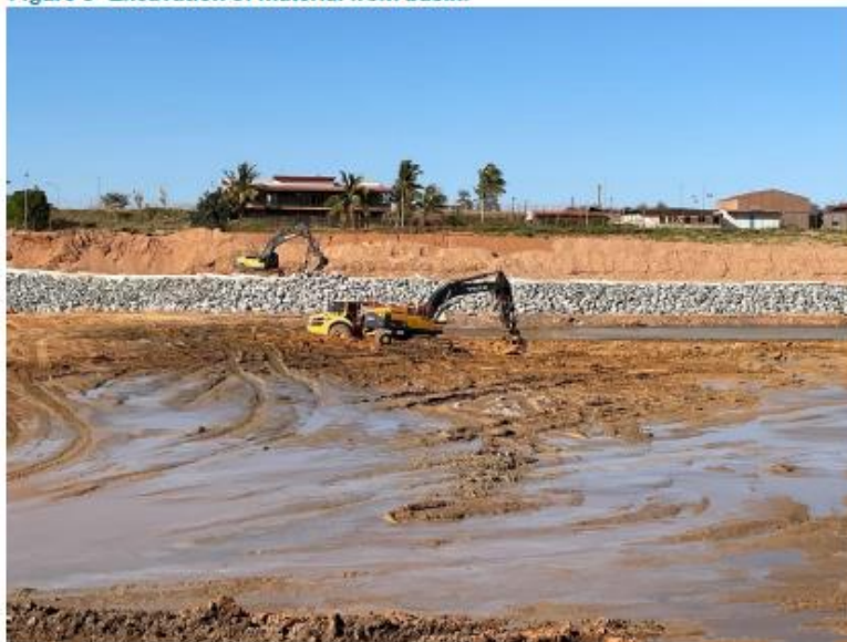
Figure 3- Excavation of material from basin.
