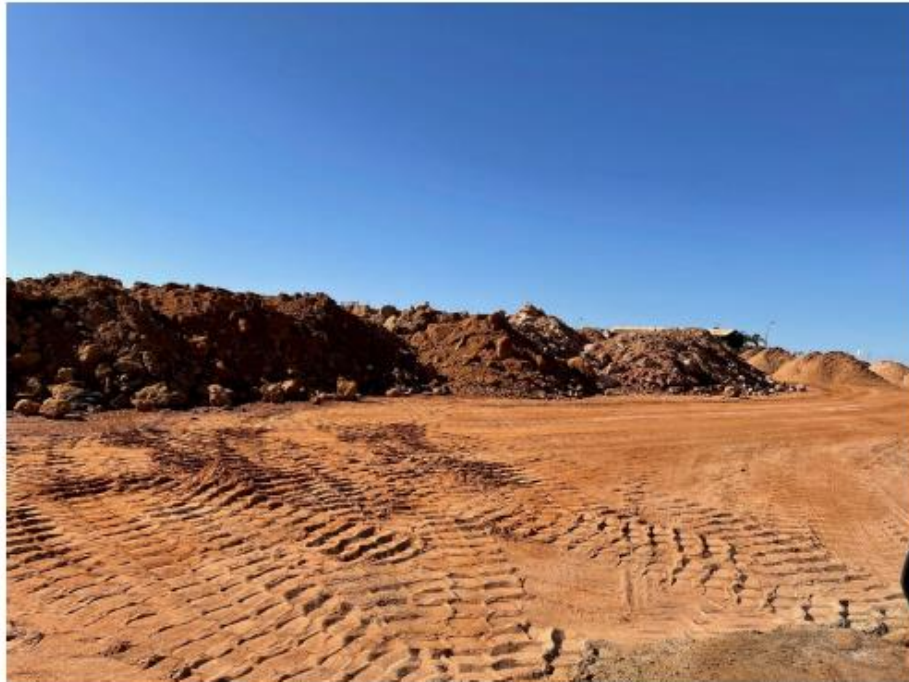
Figure 4 – Stockpiling material from basin onsite.
