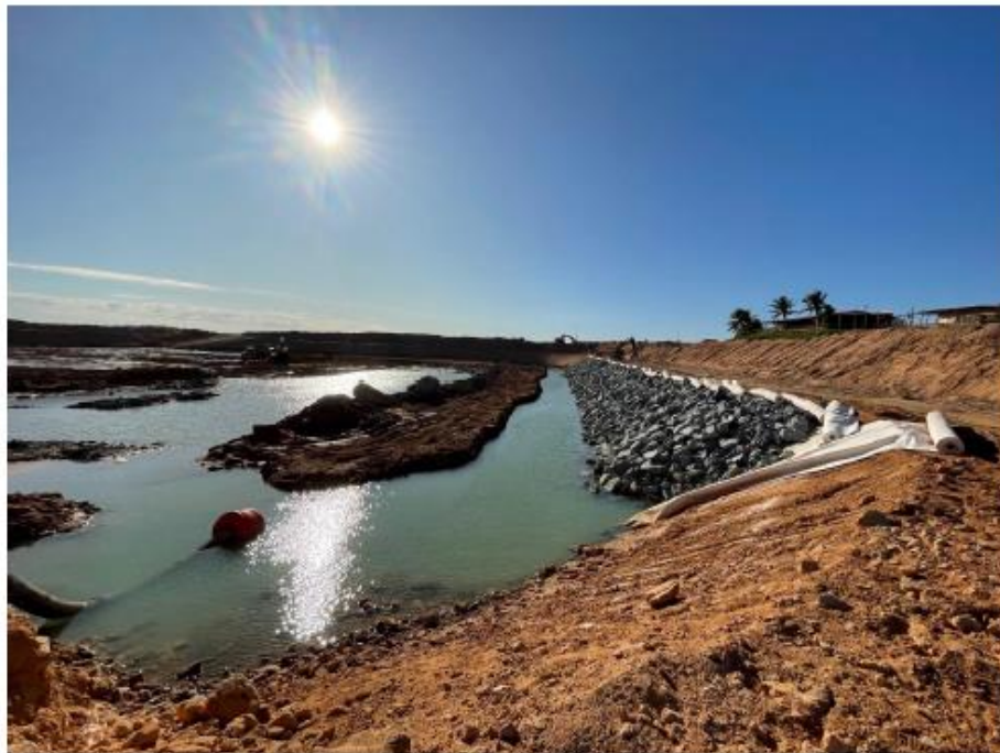
Figure 1- Rock installed across southern batter of basin.
