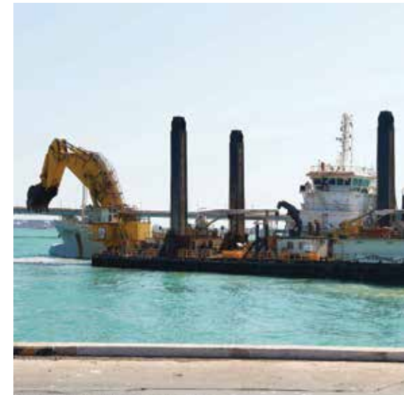
Dredging works at the HLO
