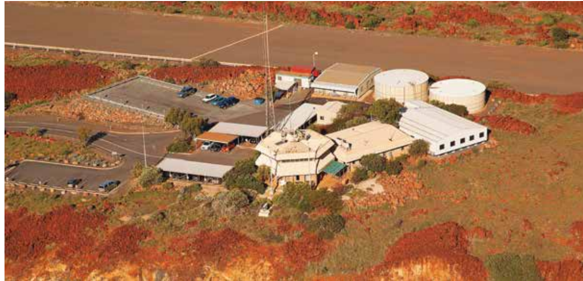
Port of Dampier communications tower and offices
