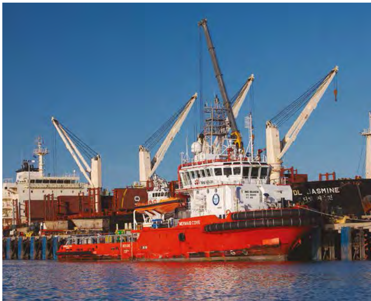
▲ Offshore supply vessel on eastern face of the Dampier Cargo Wharf
