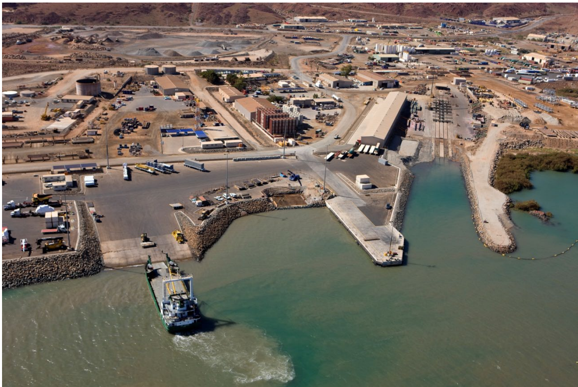
Figure 10 – Supply Base RoRo and Slipway Access
