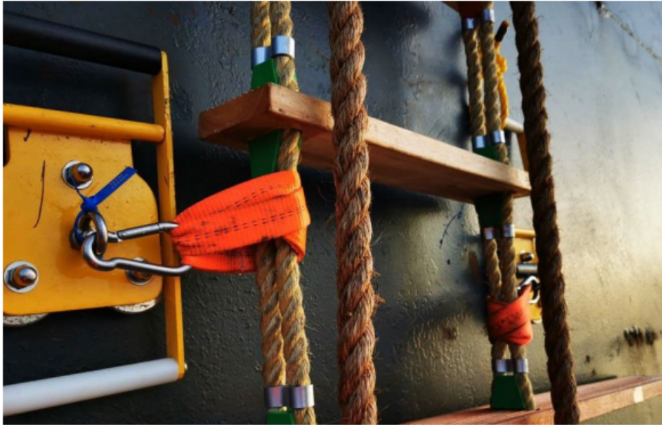
Photo 1: Example of securing both the pilot ladder and accommodation ladders with magnetic pads (Reproduced with permission from Fremantle Ports).
